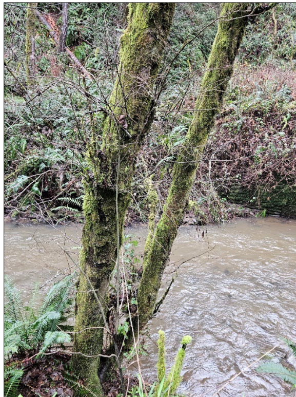
Photograph 6: View of south riverbank (just upstream of Photograph 5's vantage) where the new bridge will be constructed.
