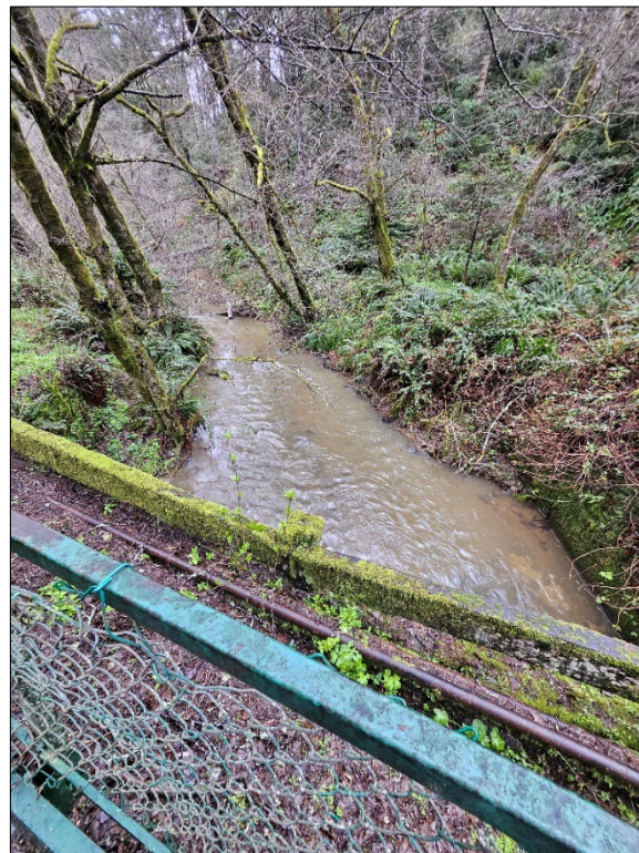
Photograph 4: View from bridge looking upstream. The replacement bridge will be placed just upstream of the existing bridge.
